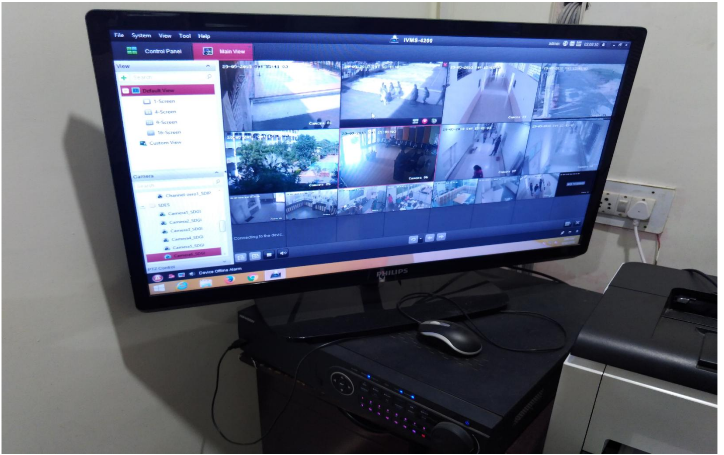
E- SURVEILLANCE FACILITY
